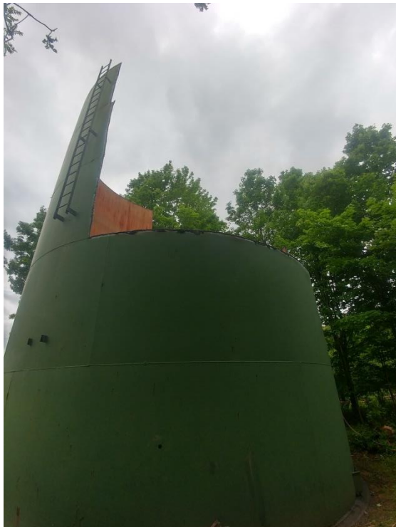
Cutting Tank Panels to Drop Inside Tank.
