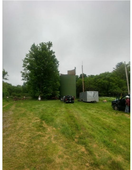
Cutting Tank Panels to Drop Inside Tank.
