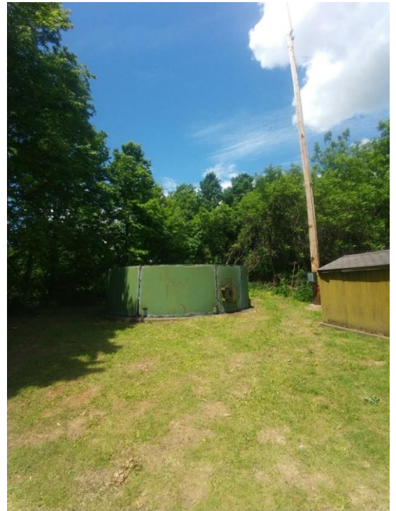
All Panels & Roof Inside Last Bottom Section Site Secured With Safety Fencing.
