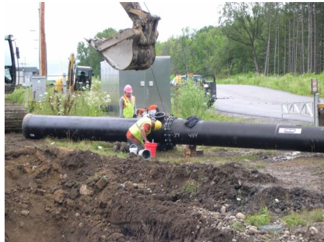
Installing 24” by EDGE’s Constructor.
