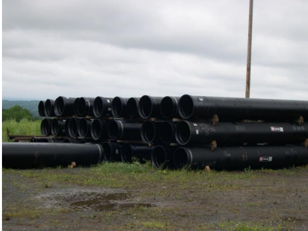
24” Pipe Stockpiled. 9,000 Feet in Total.
