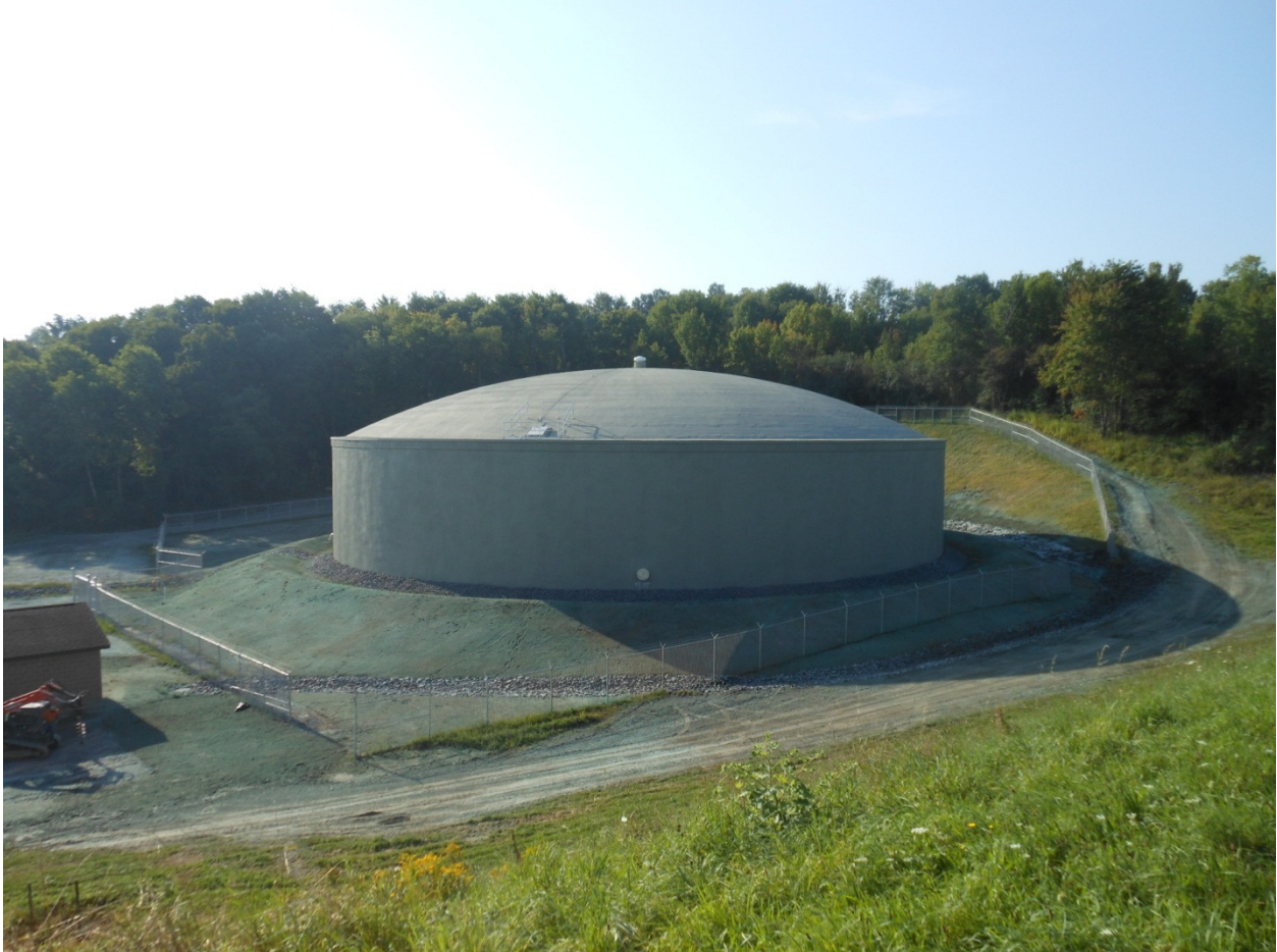
Final site Restoration – Drainage Features and Turf.
