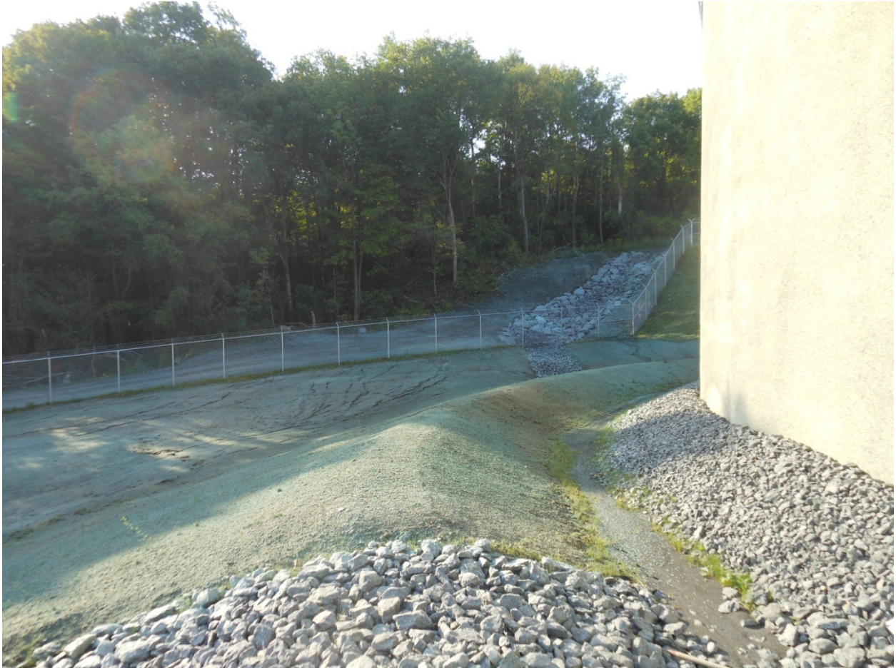
Perimeter Drainage Swales Protected With Stone Lining.
