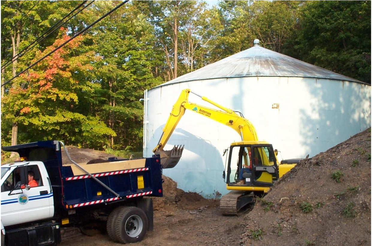
Existing Smith Hill Tank – MVWA Improved Access Several Years.
