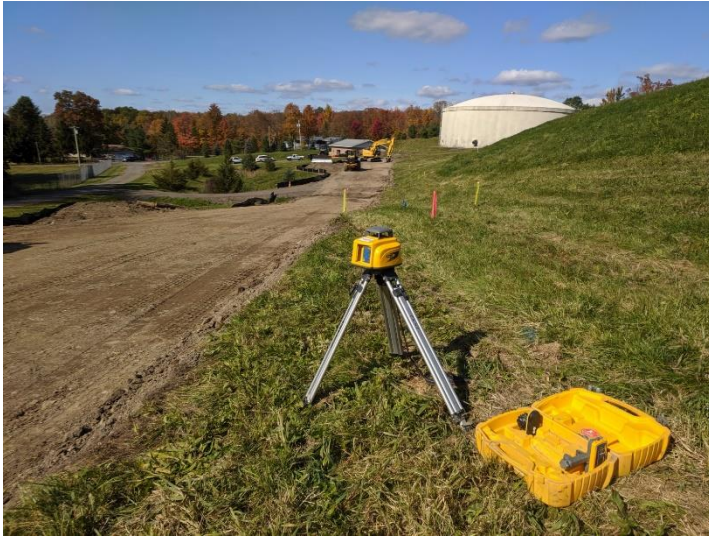
Setting Grade for Pipe Route.
