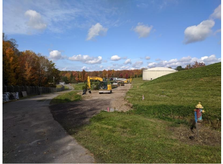
Preparing Grade for Pipe Installation.
