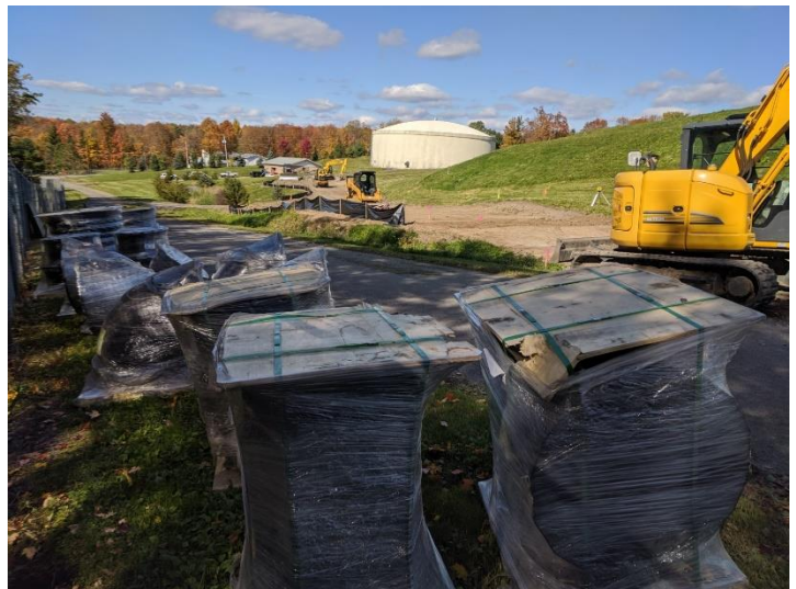
Materials Stockpile and Erosion Control Established.
