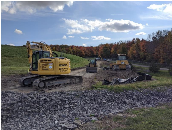
Preparing Grade for Pipe Installation.
